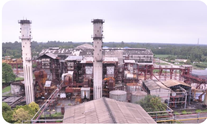
Bagasse Silos & Feeders of Boiler
