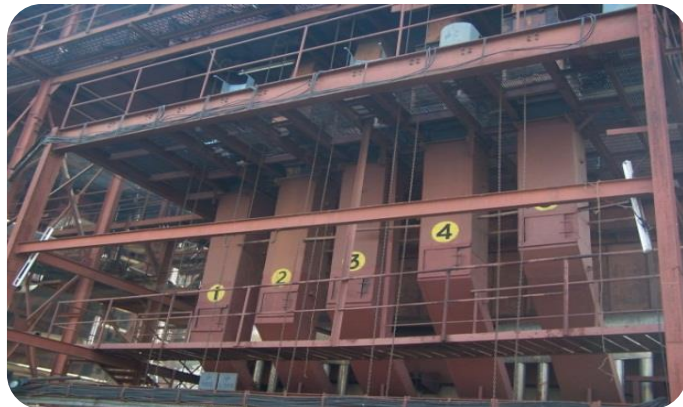
Bagasse Silos & Feeders of Boiler
