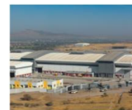
Energy Pumps Division, Shirwal
