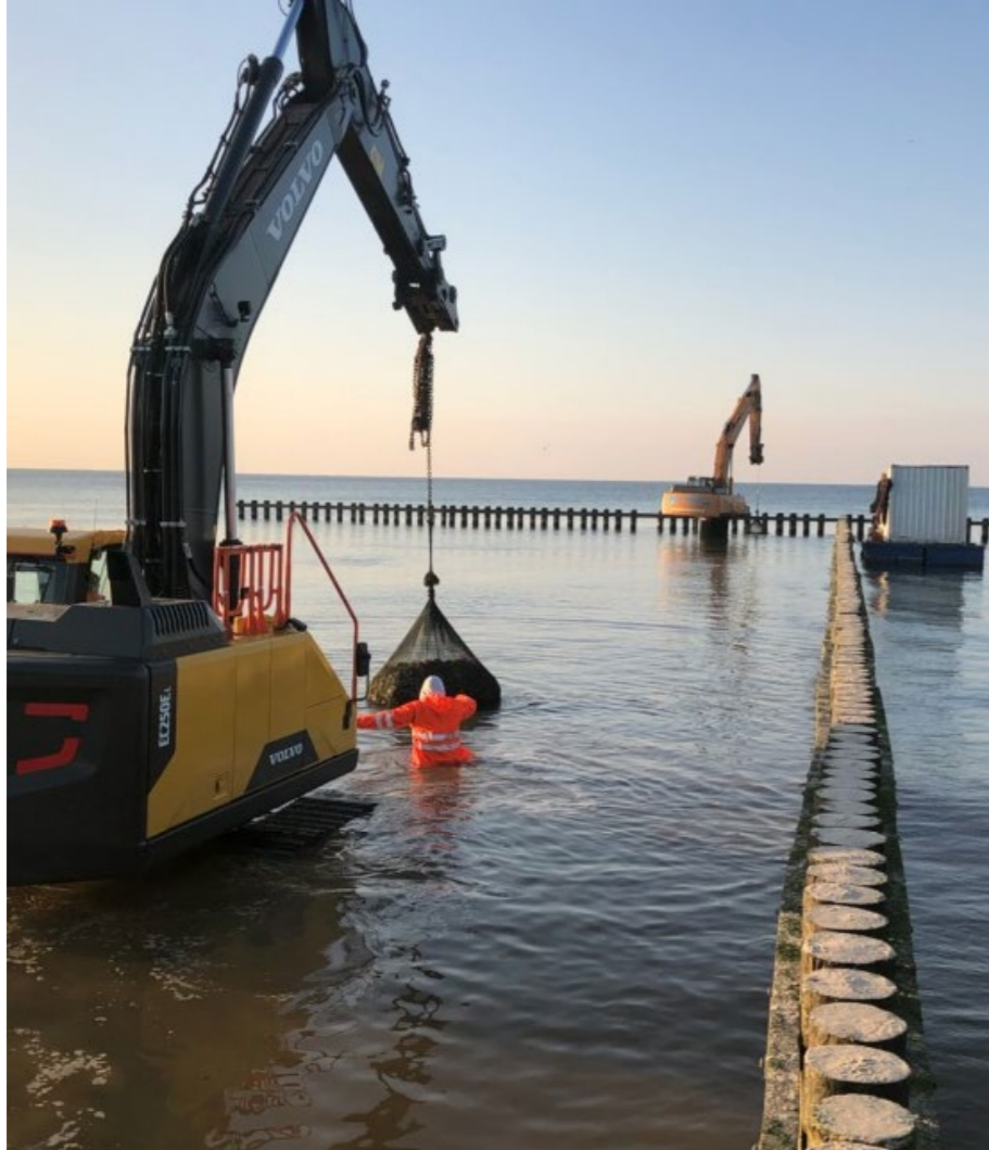
Aqua Rock Bags For Coastal Protection Works Poland
