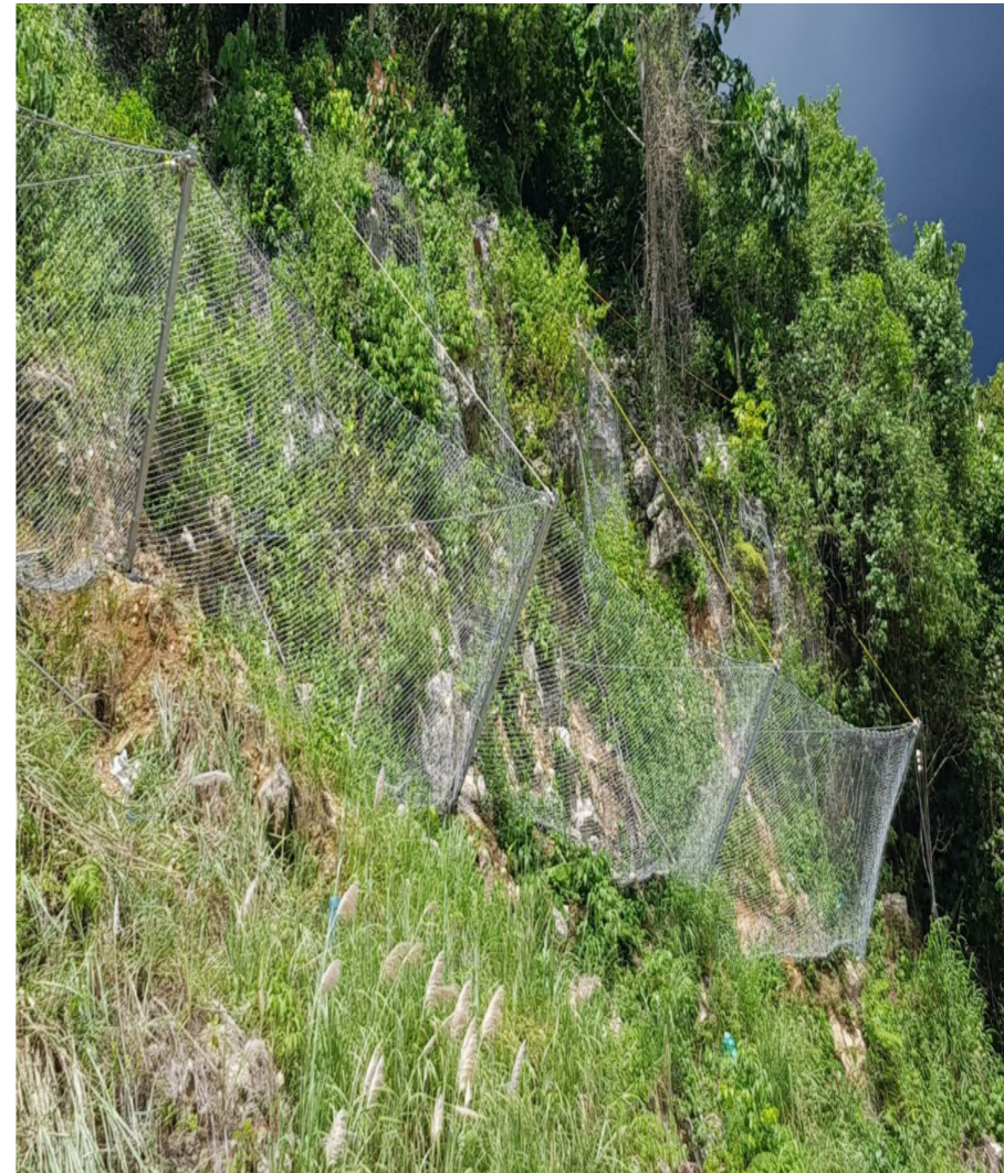
Rockfall Protection For Geohazard Mitigation Philippines
