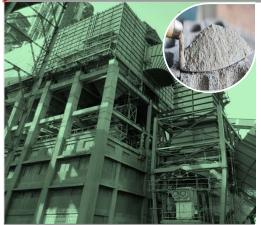
Thermax upgraded existing bag filter to RABH with 6 units of modules, addition to existing 10 units for a cement major in India.
