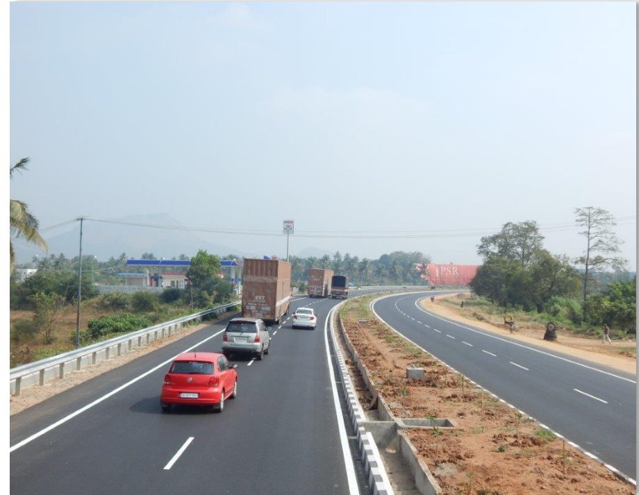
Walayar –Vadakkancherry BOT (Toll Road ) Project, Kerala
