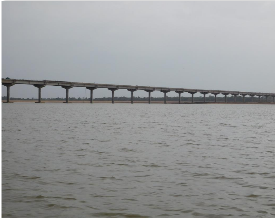
Bridge across River Godavari in Telangana State
