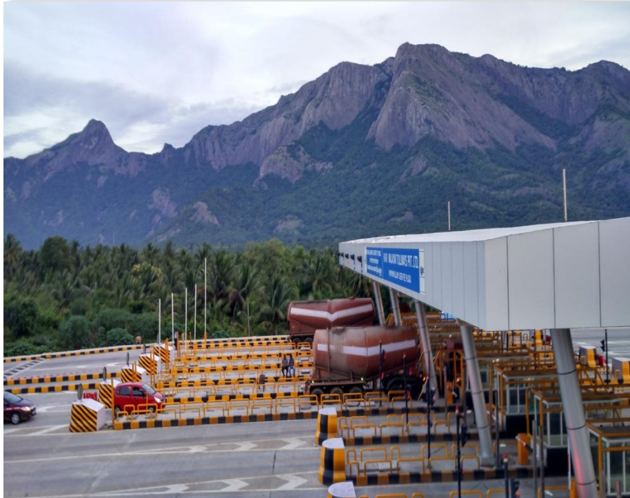
Walayar –Vadakkancherry BOT (Toll Road ) Project, Kerala
