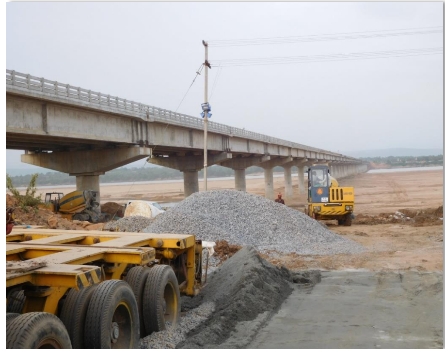
Bridge across River Godavari in Telangana State
