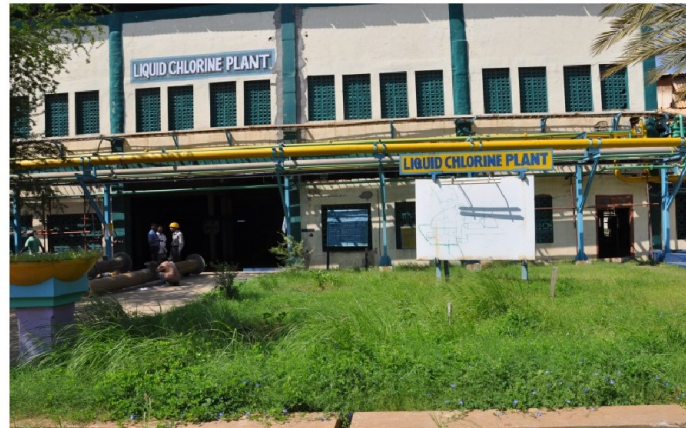
Liquid Chlorine Plant
