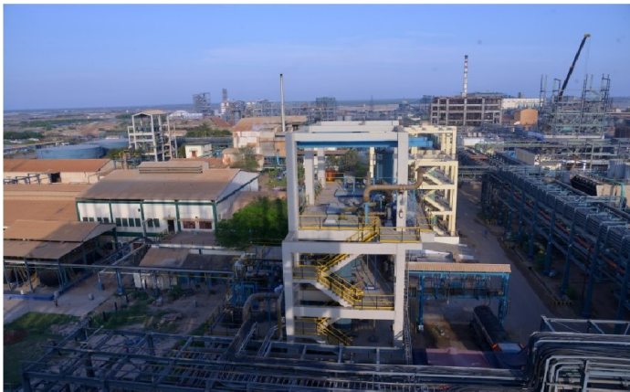
Hydrochloric Acid Plant
