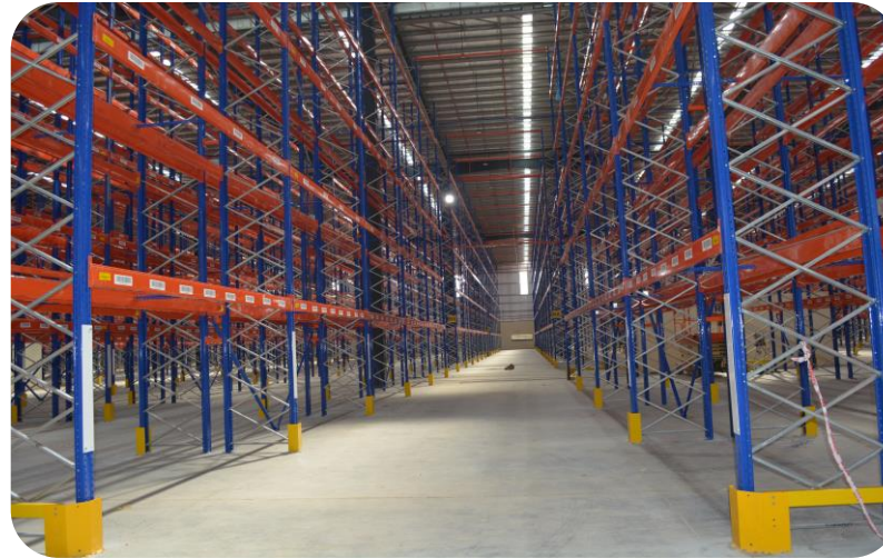
“State of the Art” infrastructure
