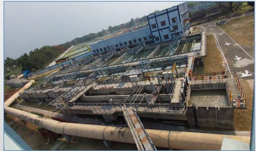
Palta WTP, West Bengal
