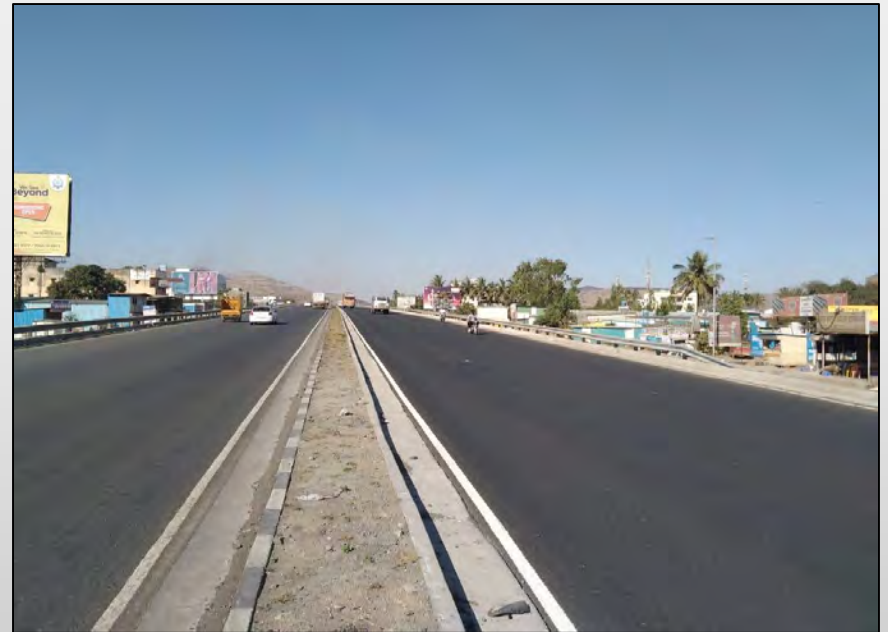
Pune Satara Road Project
