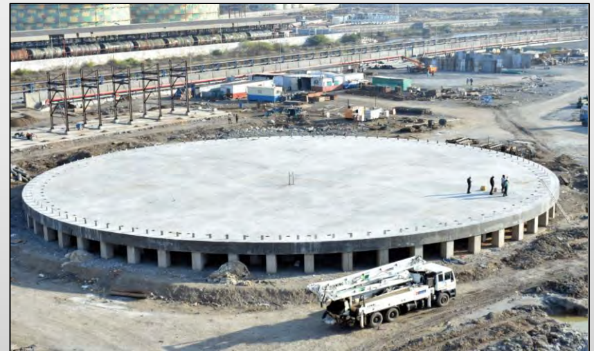
Precast Piling Project, Kandla
