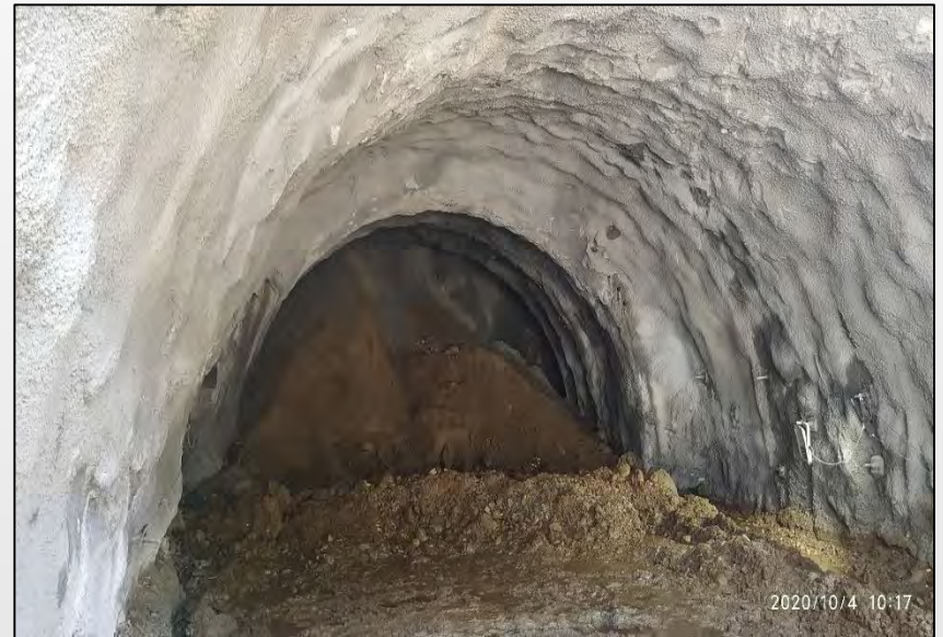
Railway Tunnel Project, Sikkim
