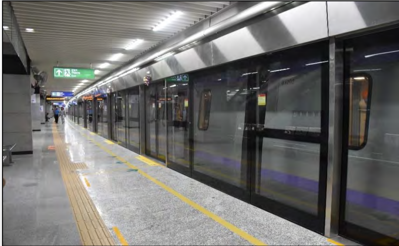
Kolkata under ground Metro Station
