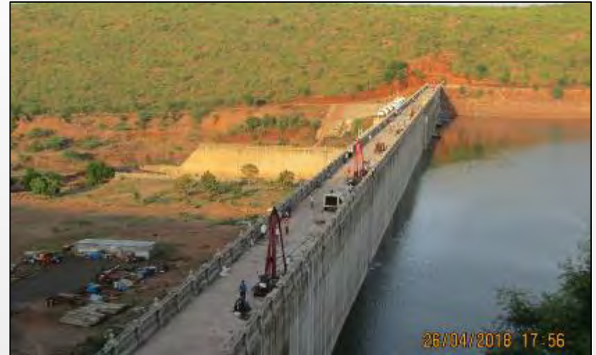
Rehabilitation of Markandeya Dam, Karnataka
