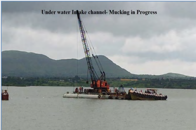
Irrigation Project, Bhama, Pune
