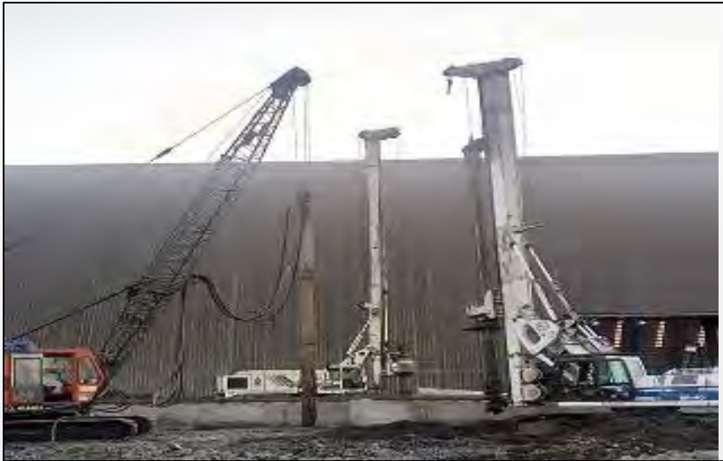
Stone Column Project, Maharashtra
