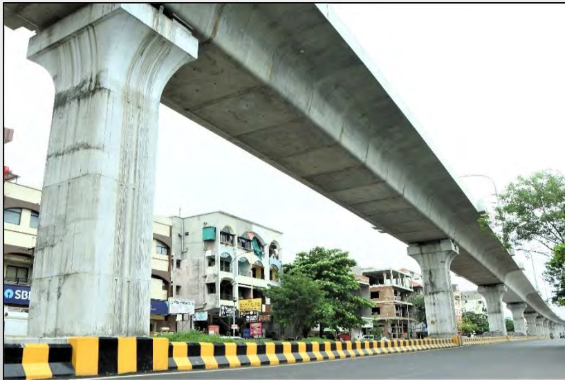
Nagpur Metro Elevated Project
