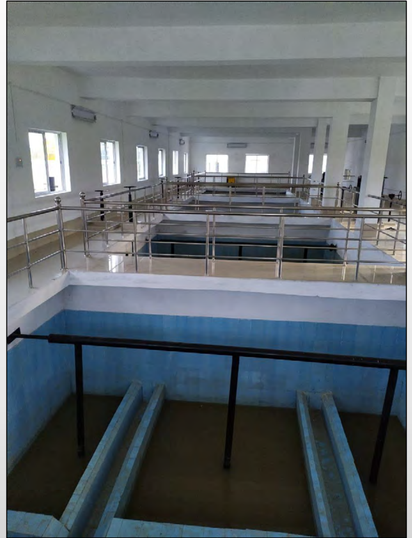
Filtration Plant at Rampur, Agartala
