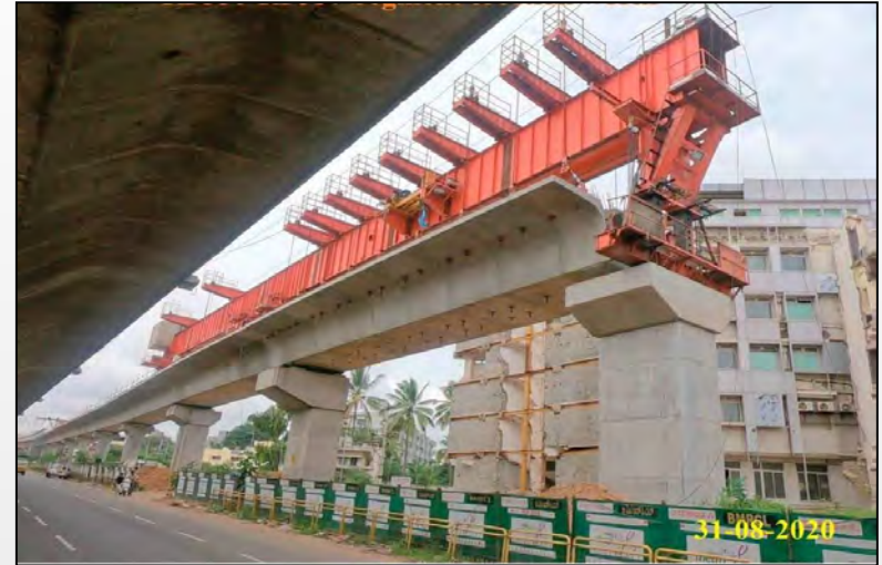
Bangalore Elevated Metro Project
