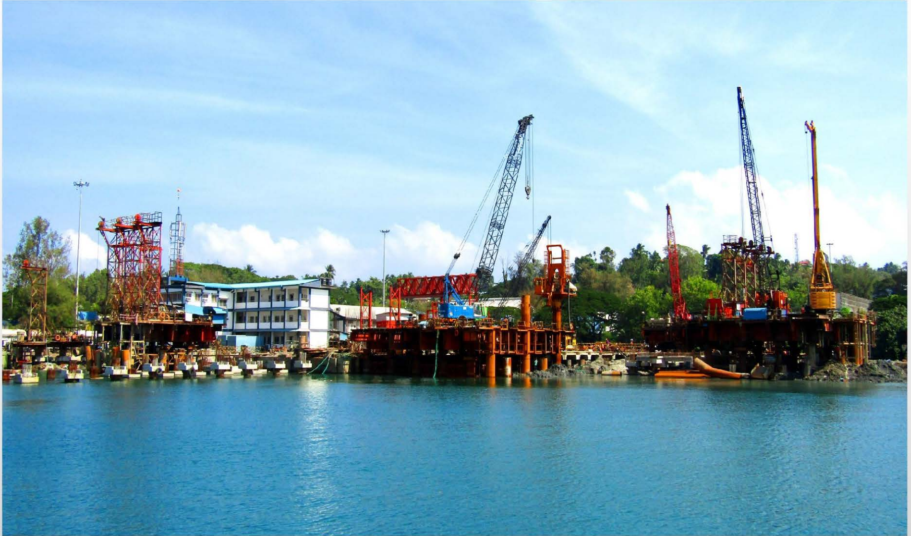
ANDAMAN LAKSHADWEEP HARBOUR WORKS , PORT BLAIR
