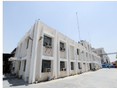
RFL I & II- Bahadurgarh
