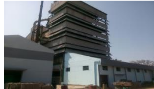
Unit 3 - New Reactive Dyes Plant
