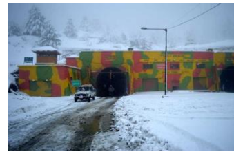
Jawahar Tunnel, J&K
