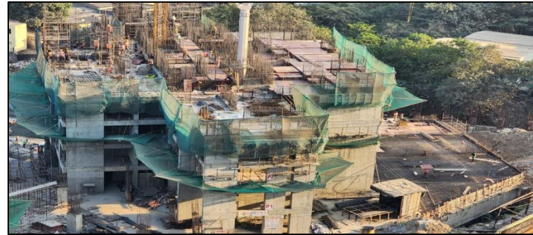
Tower B – Podium 3 slab completed
