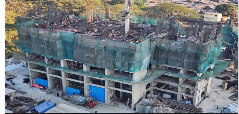
Tower A – Podium – 5 slab completed
