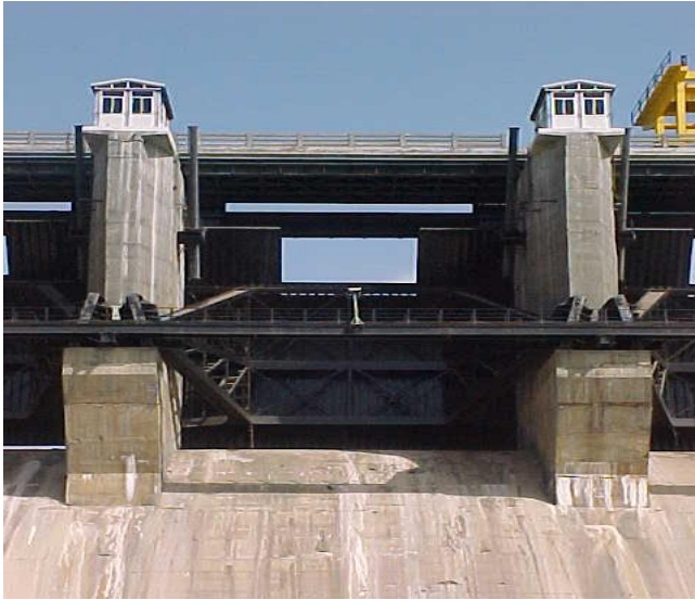
Gosikhurd Dam Client – VIDC, Maharashtra Size – 18.3m X 16.5m X 16.5m
