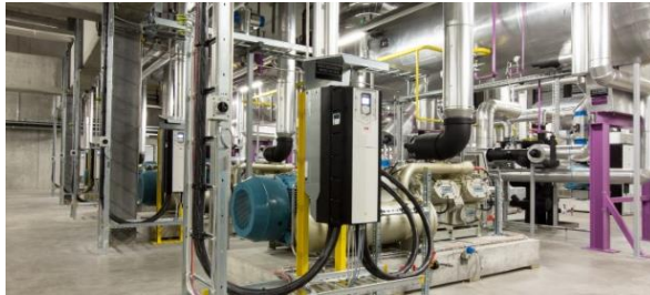
Motion solutions comprising drives and synchronous reluctance motors for heavy electricals major
