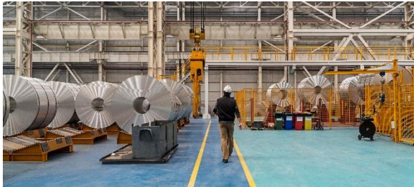
Reliable power and automation solutions for smelter and roll products for an aluminium major
