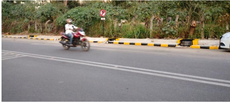
Phase-2 Peenya external road & infrastructure upgradation
