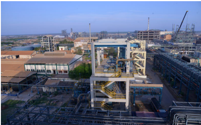
Hydrochloric Acid Plant
