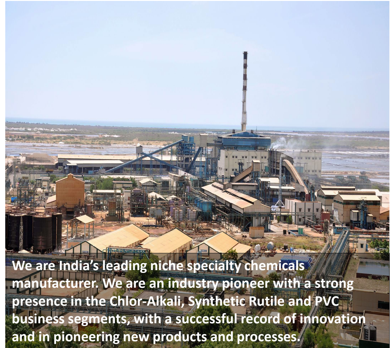
Aerial view of Sahupuram facility
