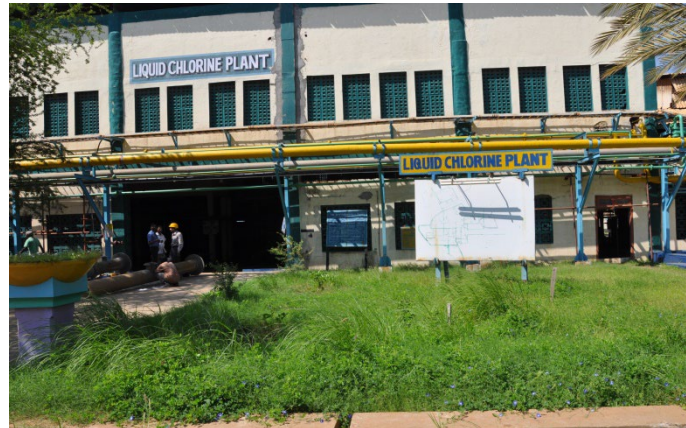
Liquid Chlorine Plant
