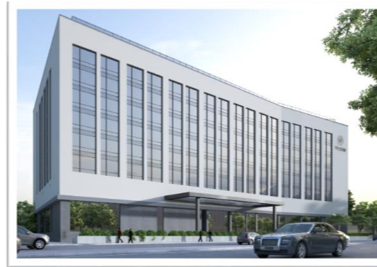
Westin 2 Hyderabad Mindspace project being evaluated with targeted opening of Q4FY23
