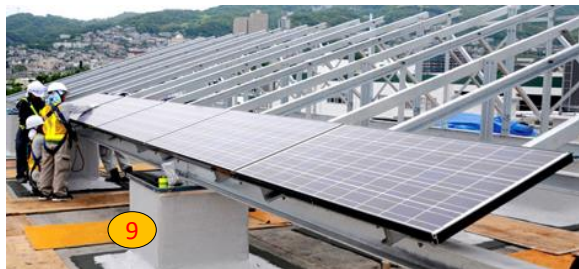
Galvalume – GL - High Strength structural steel with excellent corrosion resistance for Solar Panel structure
