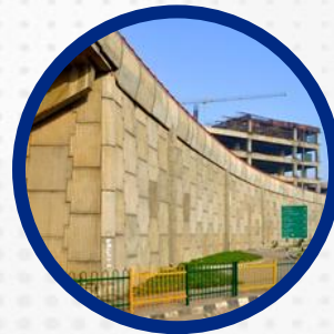
Reinforced Earth Walls
