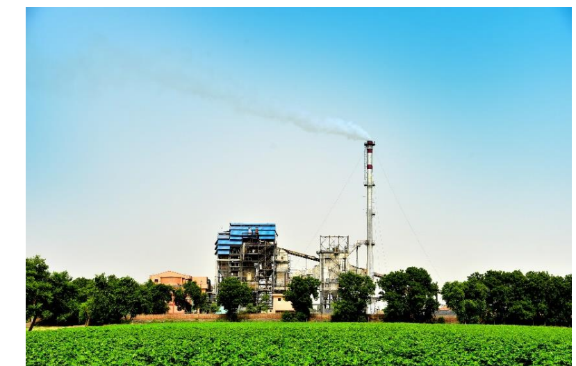
Padampur Power Plant, Rajasthan (India)
