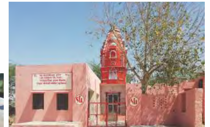
Community hall construction
