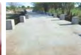
Construction of Roads
