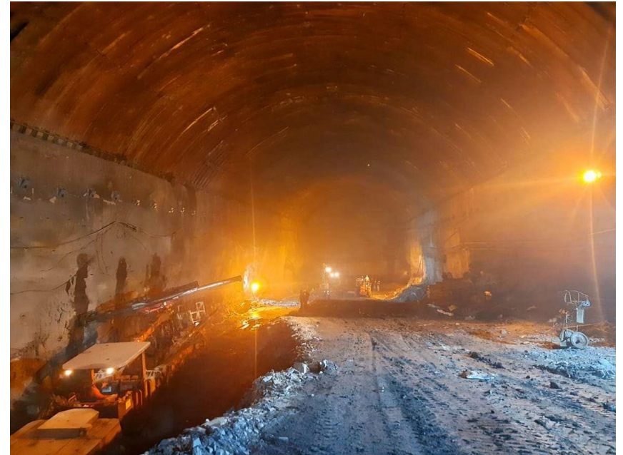
Machine Hall Benching in Progress
