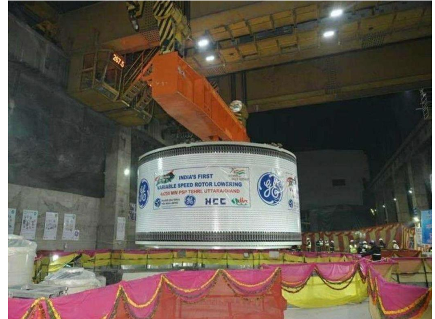
Machine Hall Unit-5 Rotor Lowering
