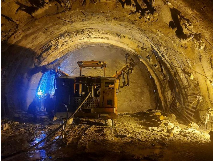
TBM Adit @ RD 238
