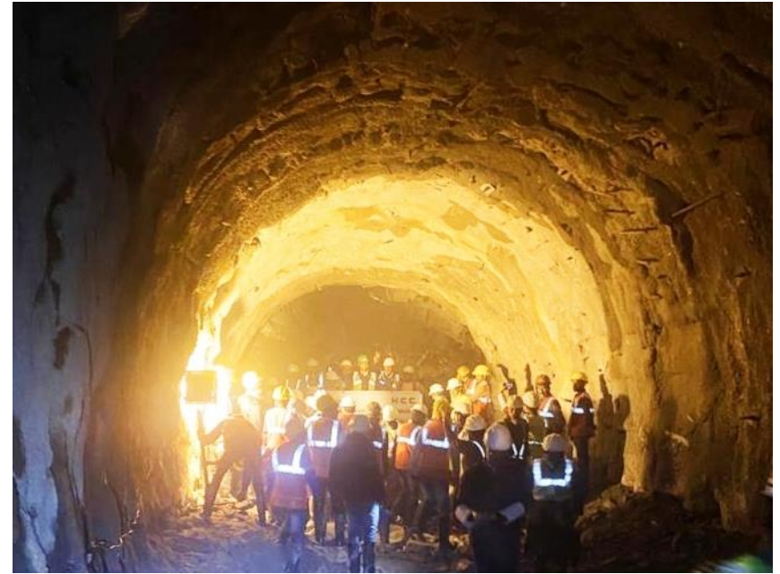
HRT Excavation completed
