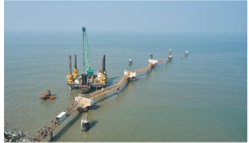
Arm 3 - Marine Piling
