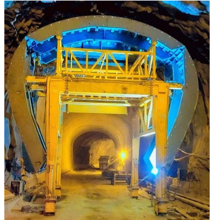
Gantry Erection at Curvature Portion
