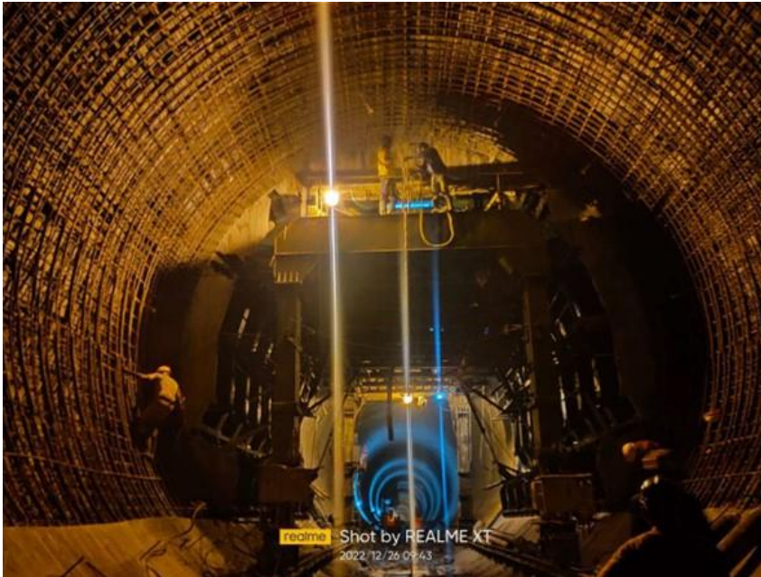
Tail Race Tunnel Reinforcement work
