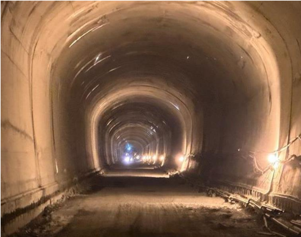
Tunnel Overt lining
