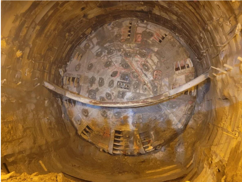
TBM Cutter Head
