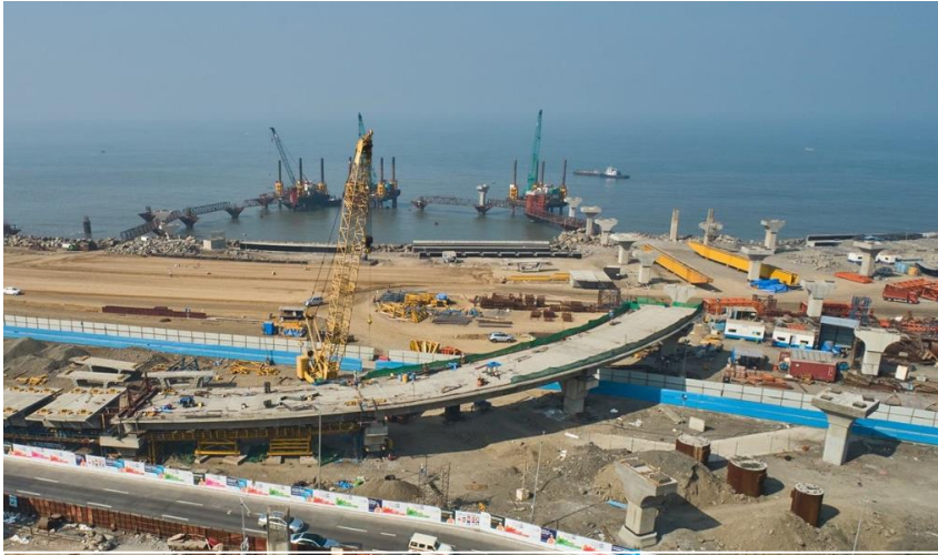
Arm 2 - Segment Erection
