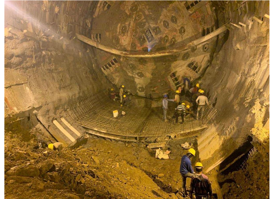
TBM Cradle Concrete
