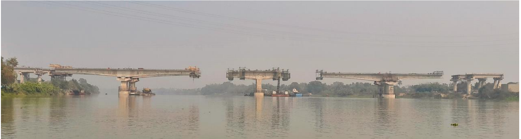
Bhagirathi bridge super structure works at Baharampore Bypass
