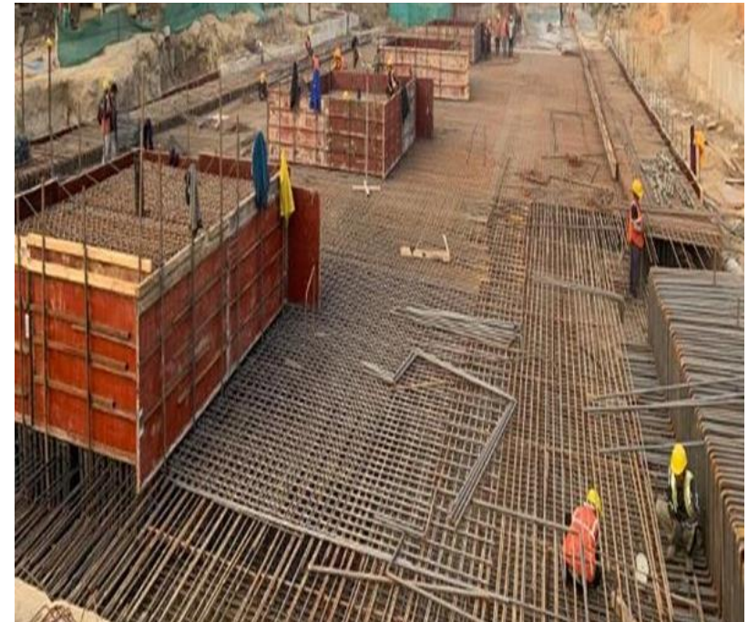
Station Roof slab in progress
