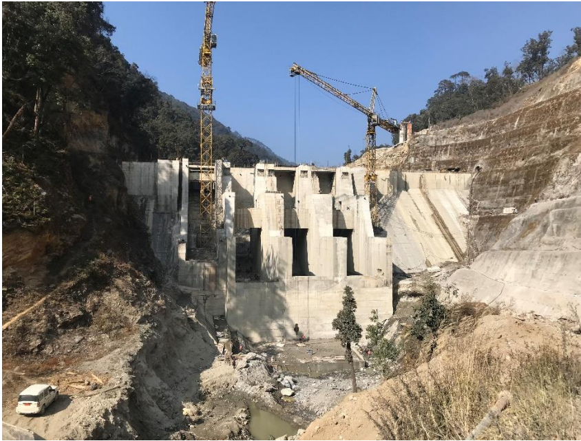
Dam works completed
