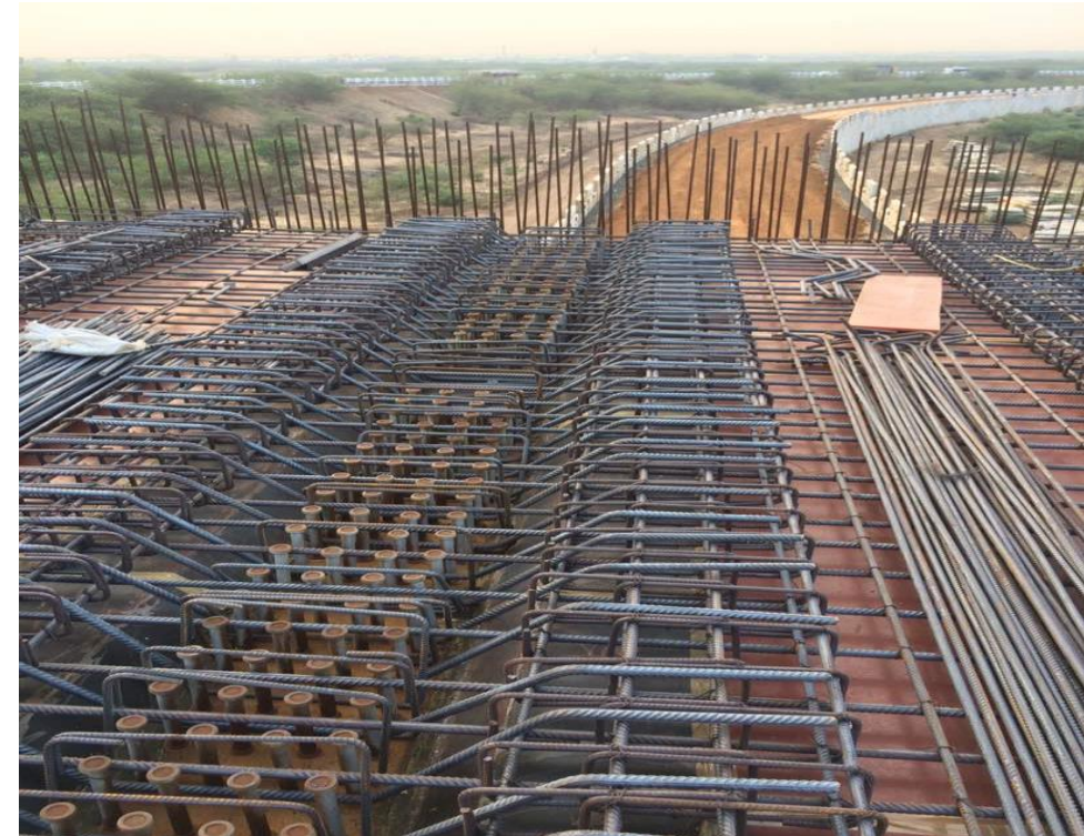
Flyover in Madurai - Ramanathpuram Section
