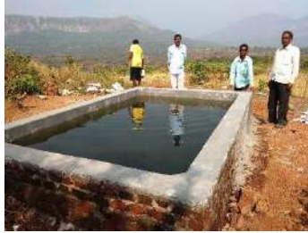
Support for water resource development and conveyance
