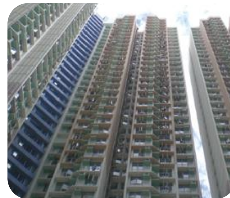
Breaking the Height Barrier
