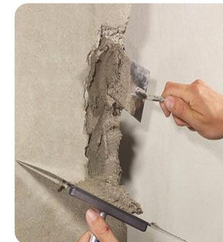
Concrete Repair, Anchors & Grouts
