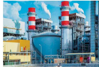
1,516 MW IBRI IPP, SEPCO – 3, Oman (Completed Project)
