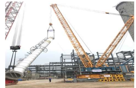
Urea Reactor Tank Installation At Ramagaundam, Telangana
