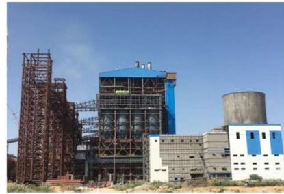
2x660 MW Suratgarh STPP, RRVUNL
