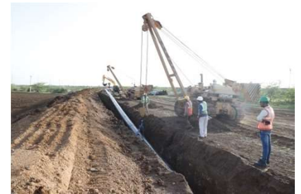
Lowering of Pipe Section, Mundra, Adani
