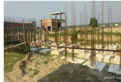
28 MLD STP at Karnal, TPL
