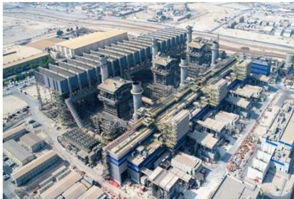
1,800 MW Alba PS5 CCPP, Bahrain (Completed Project)
