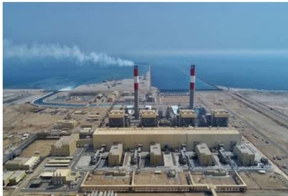
4X660 MW Shuqiaq SSPP, KSA (Completed Project)
