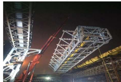
Utility Corridor, Gallery Erection, Dolvi, JSW
