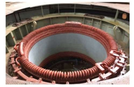
Implementation of Hydro Electric Project, 2 MW at Upper Kallar, KSEB
