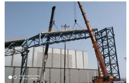
Erection of P&N Gallery at Bellary, JSW
