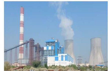
2x660 Mw STPS, Suratgrah - RRVUNL
