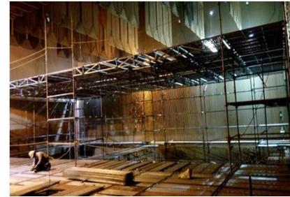
Cuplock Scaffolding Erection 800 MW, Mundra
