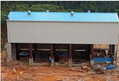
Implementation of Hydro Electric Project (2MW/5.14 Mu)-KSEB
