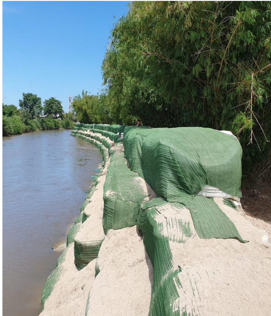
Fabric Forms (Geo-containers) For River Training Works Colombia
