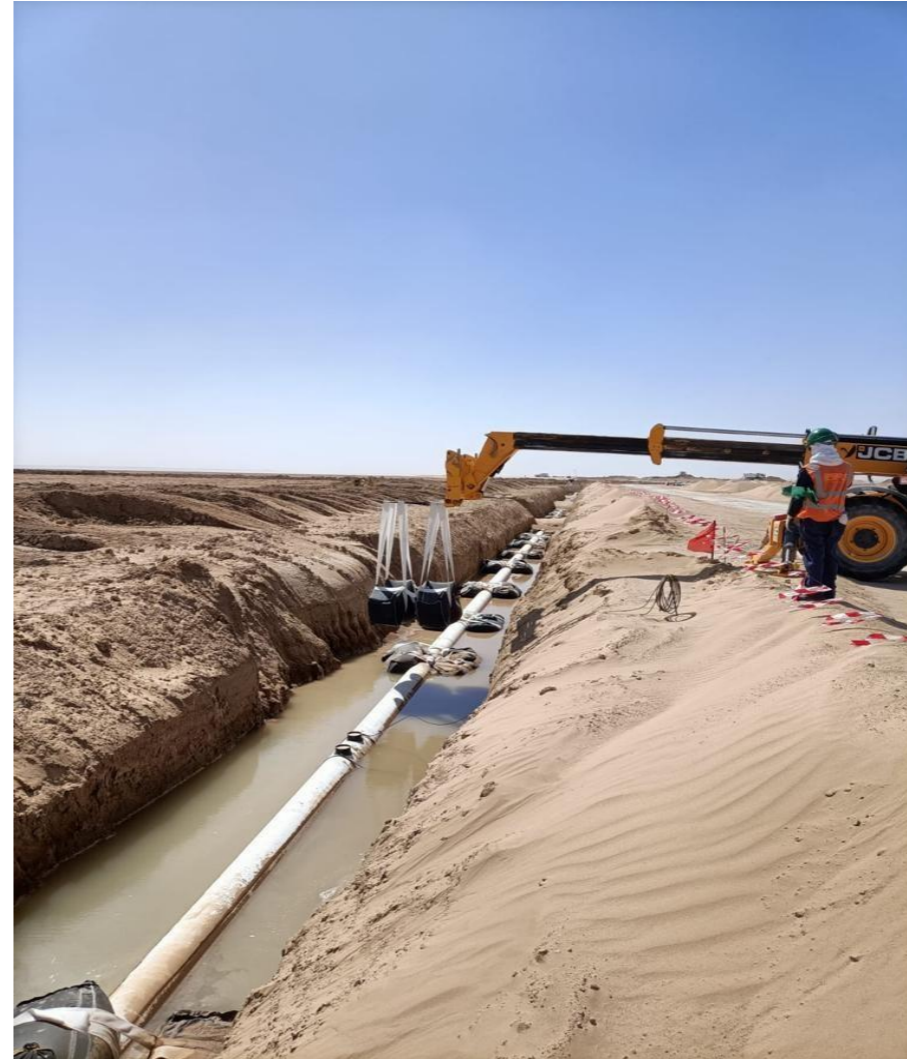
Fabric Forms (Saddle Bags) For Pipeline Protection Works Oman
