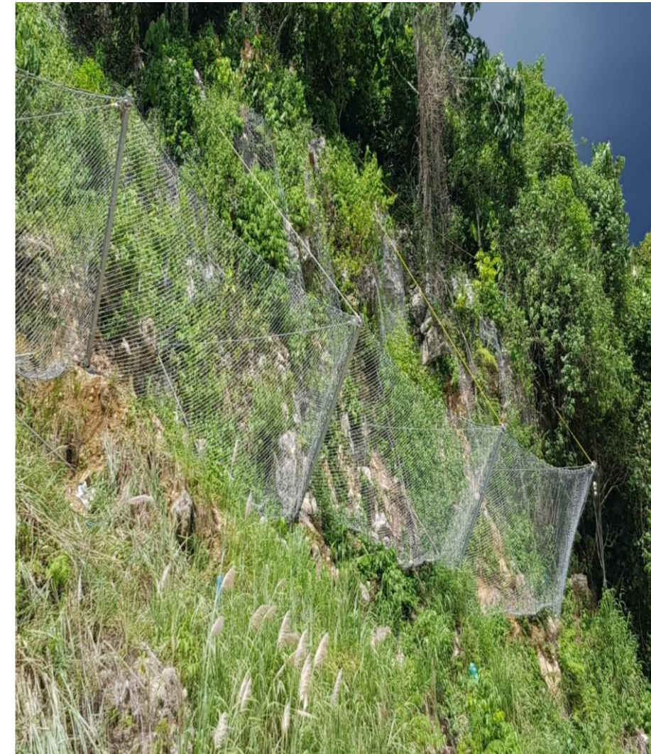
Rockfall Protection For Geohazard Mitigation Philippines
