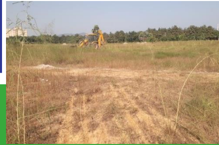
78MWp groundmount Project at Tamnar, Chhattisgarh
