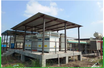
154MWp ground mounted project at Thoothukudi, Tamil Nadu
