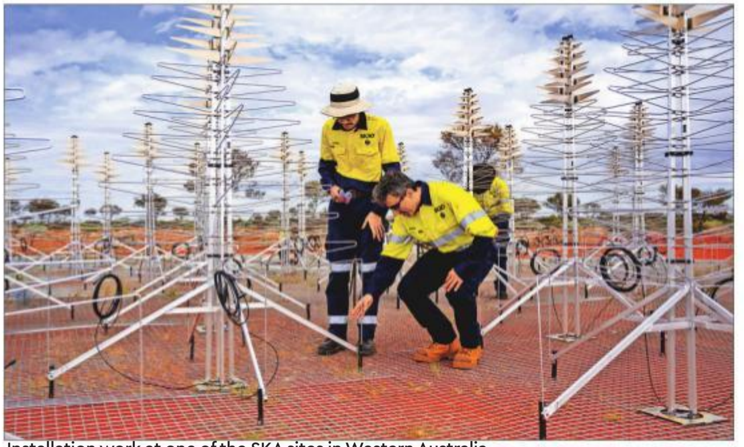
Installation work at one of the SKA sites in Western Australia.
