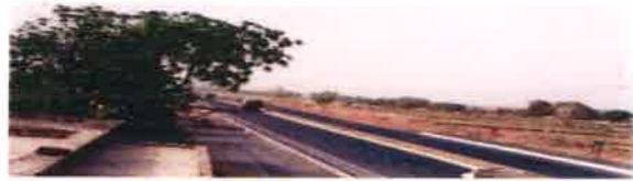
Project: Four laning of NSEW corridor of Agra Dholpur section of NH-3
