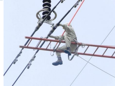
Hot line maintenance work
