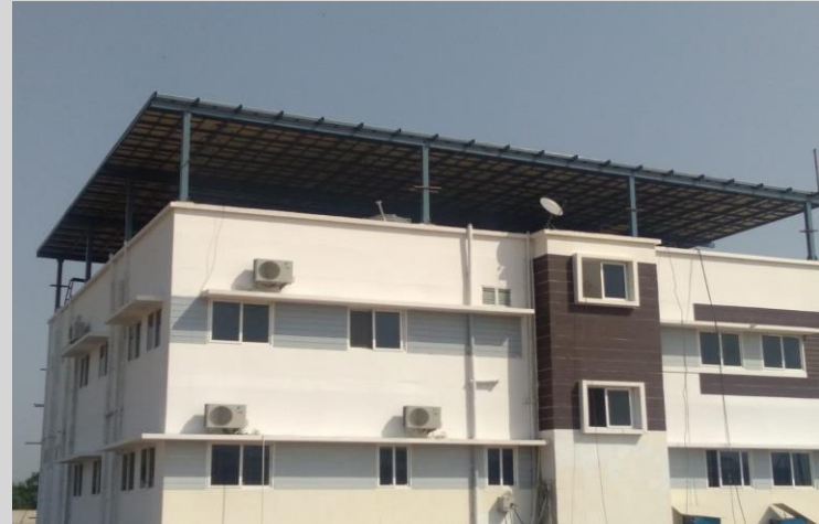
ROOFING WITH THE ATUM PANELS
