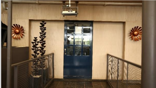
Wall Paneling with V-Boards
