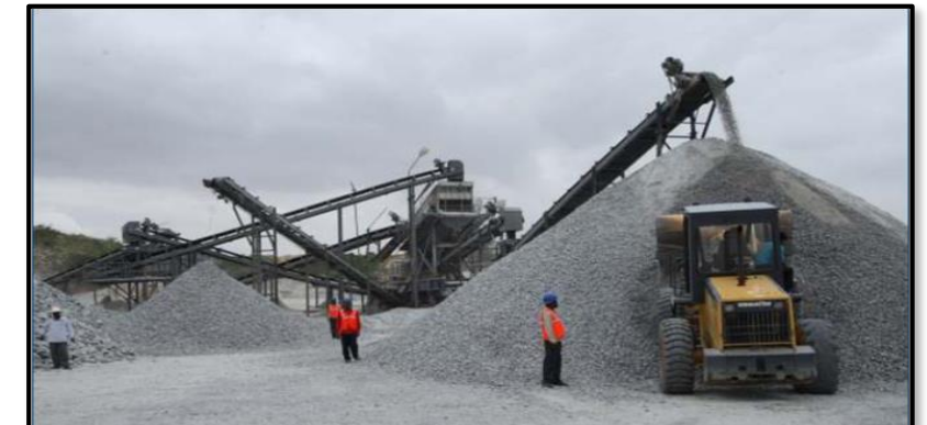
250 TPH Nawa Crushing Plant
