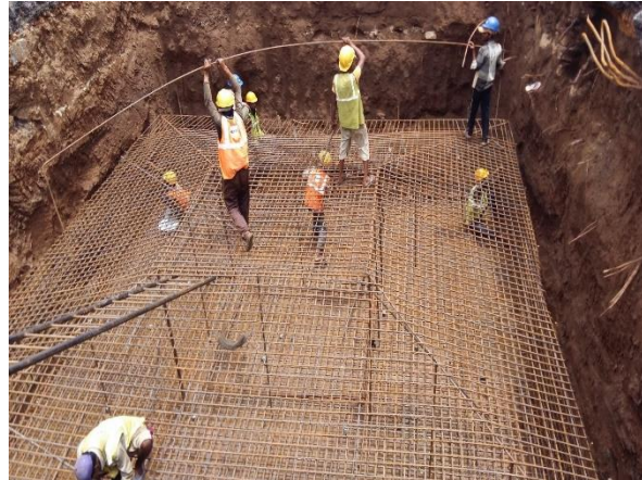
Workers on Site
