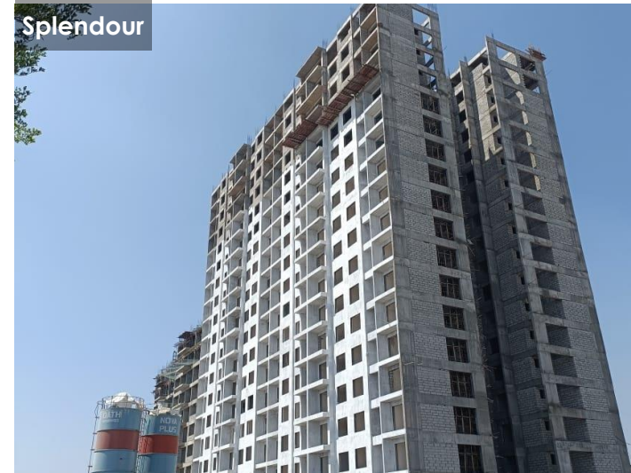
Project Status as on Sep 2023
