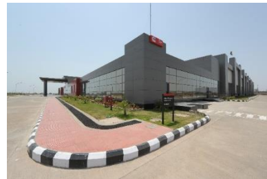
Tata Cummins plant II Phaltan
