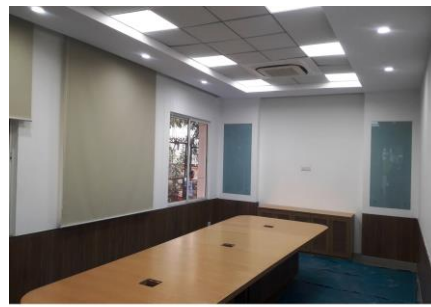
Wall Cladding & False Ceiling
