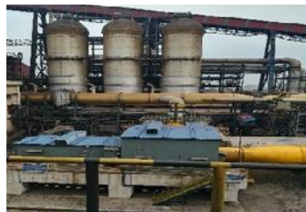
BLAST FURNACE, STEEL PLANT WORK, JSPL, ANGUL
