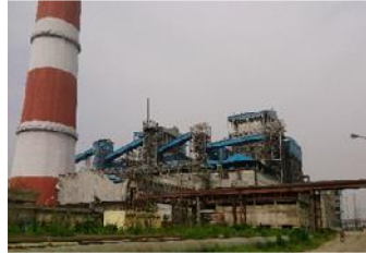
2X500 MW STPP,BOILER, ESP STG, VINDHYACHAL, BHEL (COMPLETED)
