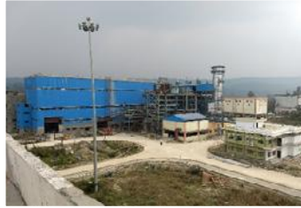
1X100 MW CCPP, BALANCE CIVIL & STRUCTURAL WORKS, NAMRUP, BHEL (COMPLETED)
