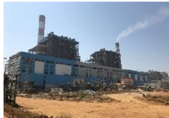
2X660 MW IBTPS, STRUCTURE & STG, BANHARPALLI, BHEL
