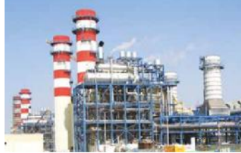
2X157 MW GT POWER PLANT, LIBYA (COMPLETED)
