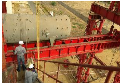
HP HEATER REPLACEMENT 800MW ,CGPL MUNDRA2
