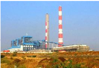
3X800 MW, BOILER, ESP, PIPING, STG KUDGI , DOOSAN, L&T & TOSHIBA
