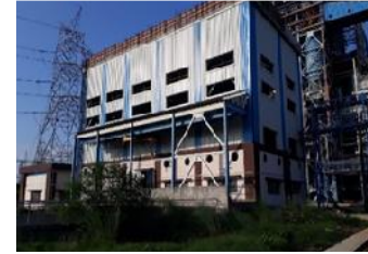
1X500MW, FGUTTP, CIVIL, STRUCTURAL AND ARCHITECTURAL WORK FOR BTP, BOP & CHP, UNCHAHAR, NBPL
