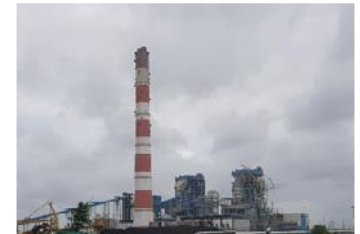
2X660 MW STPP, BOILER, ESP U#1&2, SOLAPUR, BGRESL
