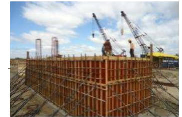
1X110 MW, CIVIL AND STRUCTURAL WORKS ,R&M OF MAIN PLANT, BATHINDA, BHEL
