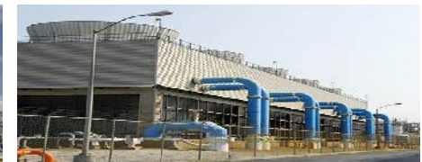
Infrastructure Construction (Civil)
