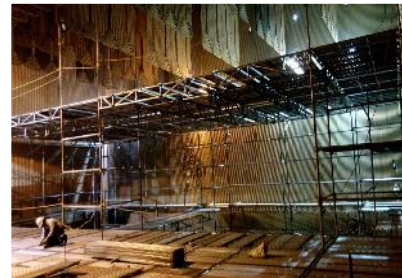
CUPLOCK SCAFFOLDING ERECTION 800MW,MUNDRA
