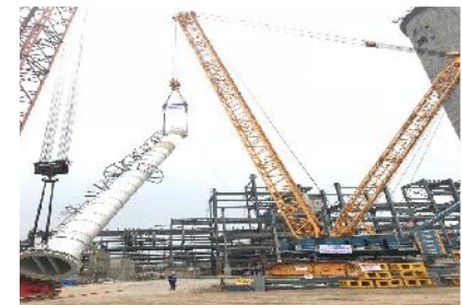
UREA REACTOR TANK INSTALLATION AT RAMAGAUNDAM, TELANGANA
