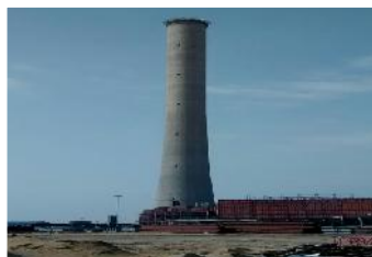
1X500 MW, FGUTTP, CIVIL, STRUCTURAL AND BOP & CHP, UNCHAHAR, NBPL
