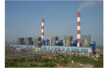
BOILER, ESP, STRUCTURE, TG AUXILIARIES,UMPP 6X660MW, SASAN, R INFRA (COMPLETED)
