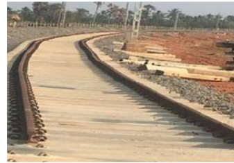
GDV-MTM 37 ,DOUBLING & ELECTRIFICATION WORKS , RVNL
