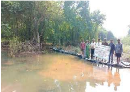
Check Dam: Moravane, Chiplun, Ratnagiri
