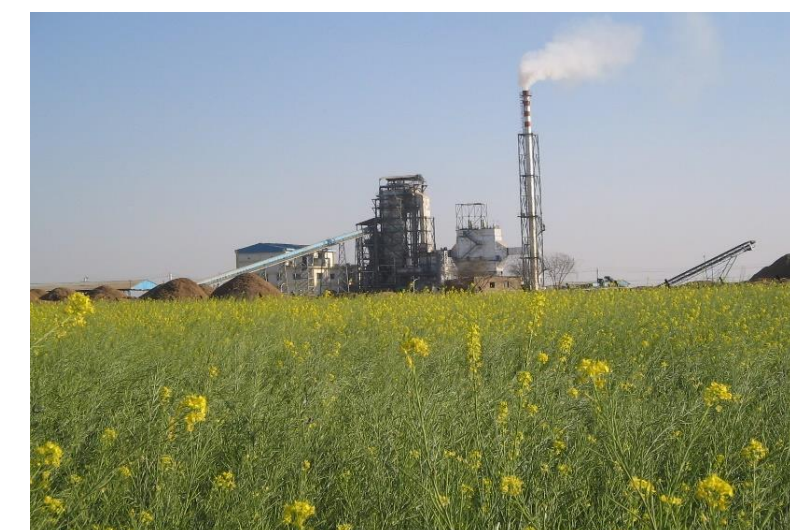
Uniara Power Plant, Rajasthan (India)
