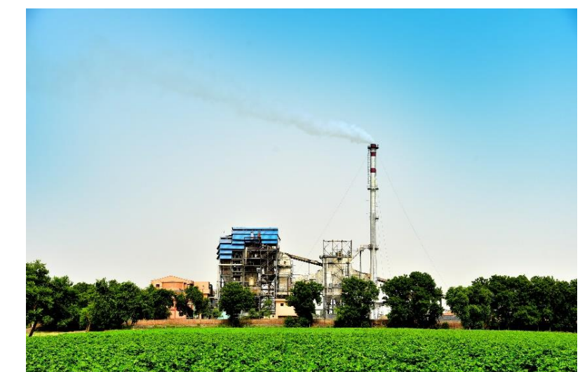
Padampur Power Plant, Rajasthan (India)
