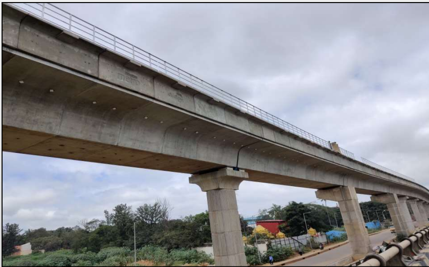
Bangalore Metro Elevated Project
