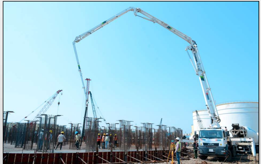
Precast Piling Project, Kandla
