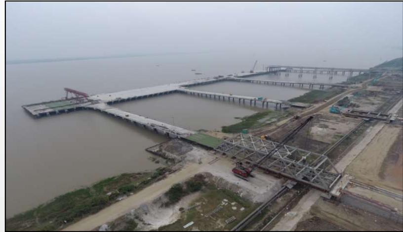
Haldia Inland Waterways Jetty
