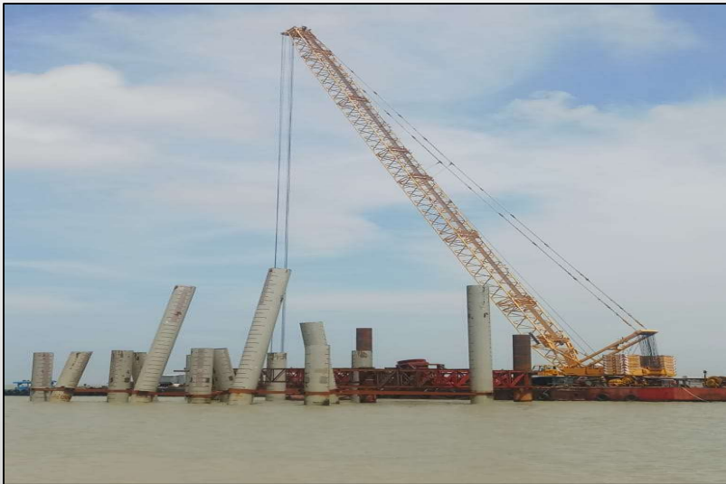
Dhamra Orissa Steel Piling Project
