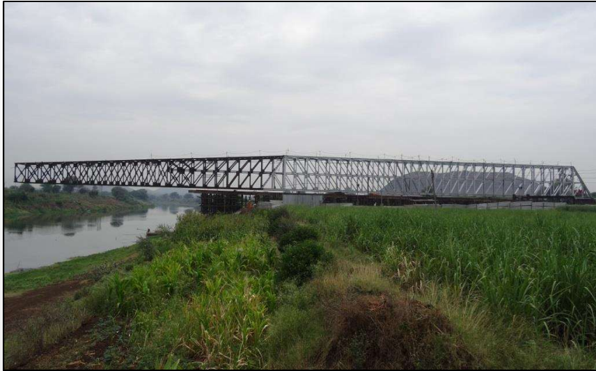
Dharna Bridge, Nashik
