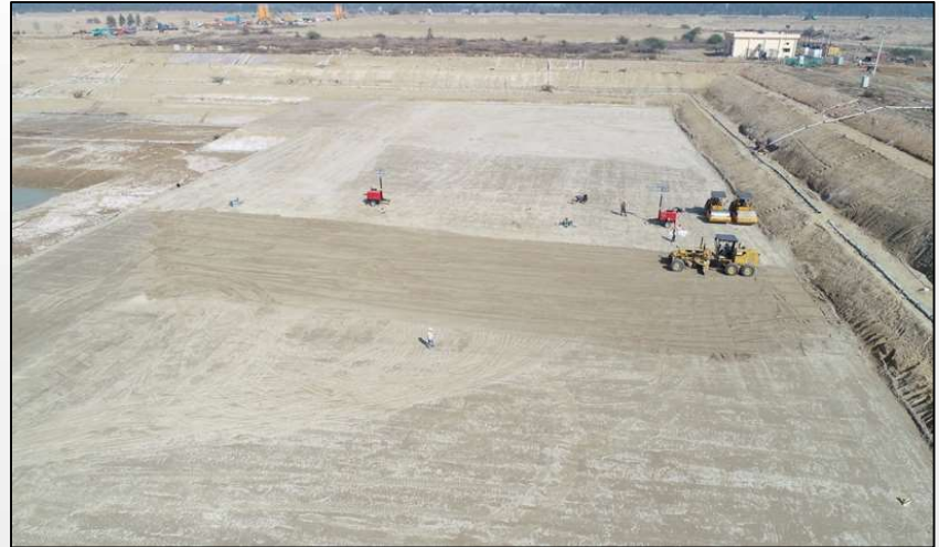
Ground Stabilization work, Haryana
