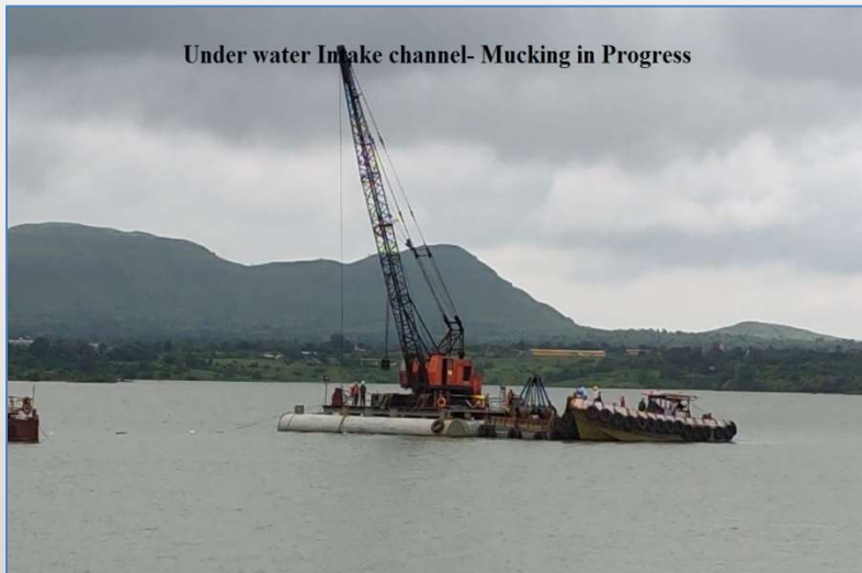
Irrigation Project, Bhama, Pune
