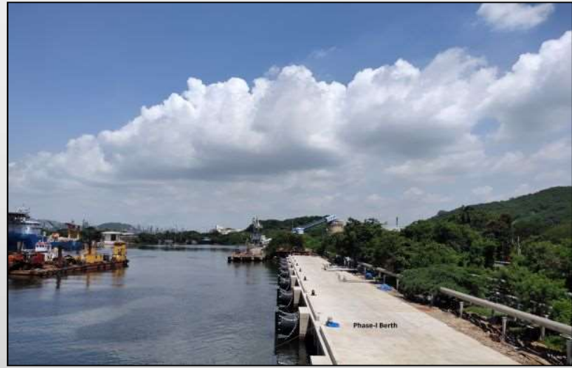
Vizag Port Marine Jetty
