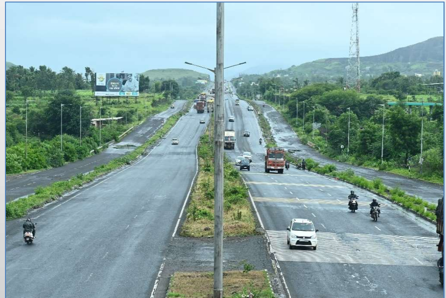
Pune Satara Road Project
