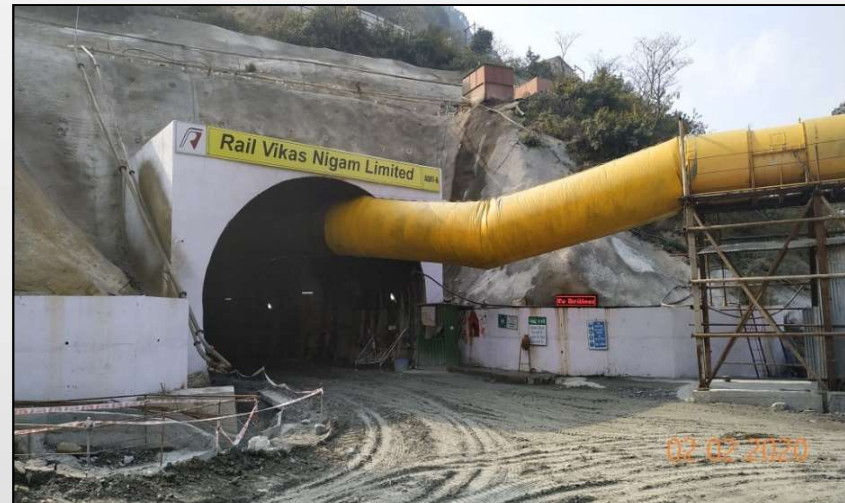
RVNL Tunnel Project, Uttarakhand
