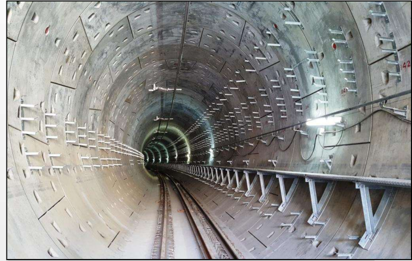
Mumbai Metro Underground Tunneling Project
