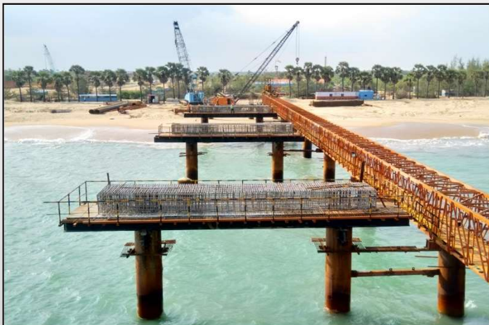
Udangudi Power Project – Piling Work
