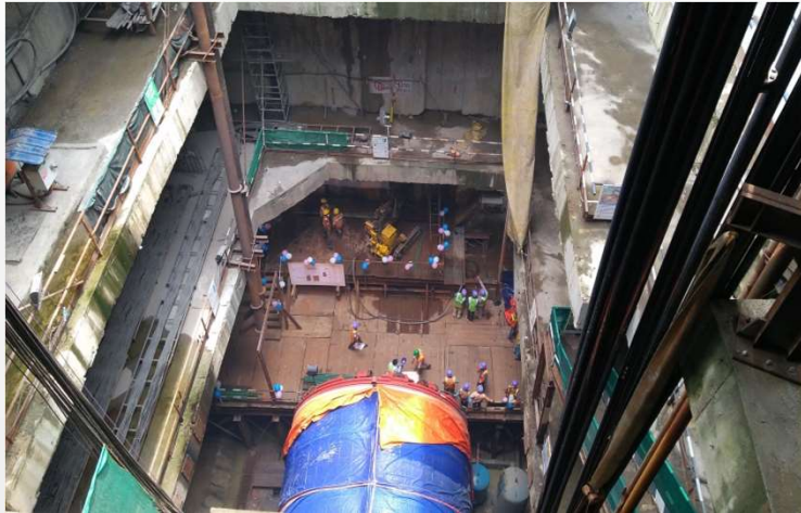
Underground Kolkata Metro Project
