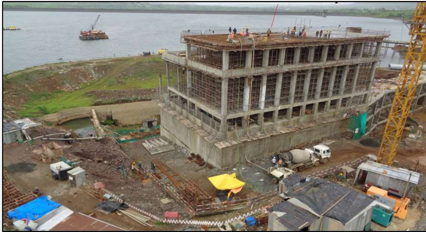
Bhama Ashed Water Supply Project
