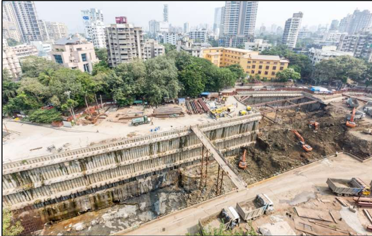
Secant Piling at Siddhivinayak Station for Mumbai Underground Metro Project
