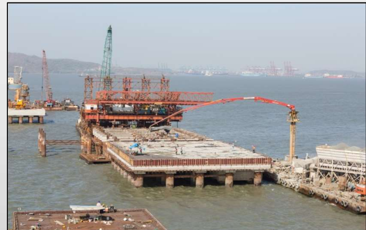
Mumbai Port Trust Project
