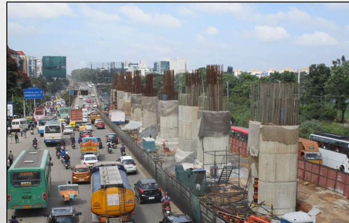
Bangalore Metro Project
