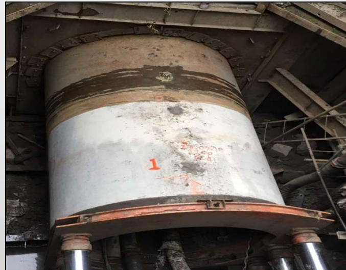
Micro Tunneling at Kolkata
