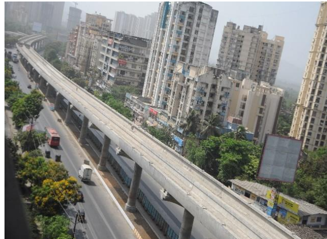
Mumbai Metro Line 4A
