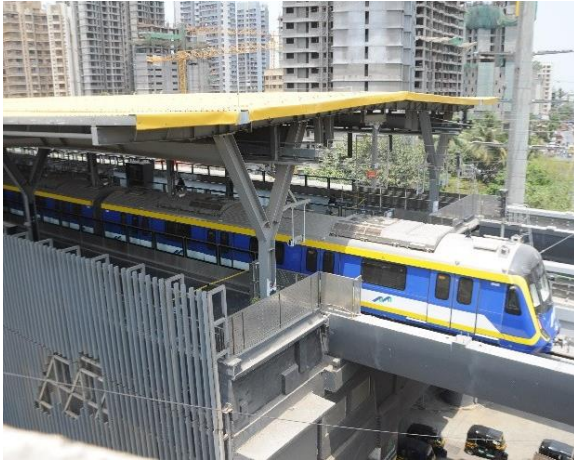
Mumbai Metro Line 2A
