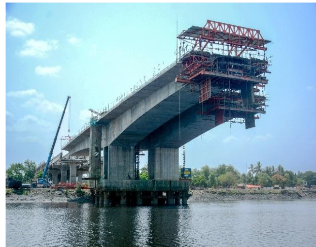
Motagaon Creek Bridge
