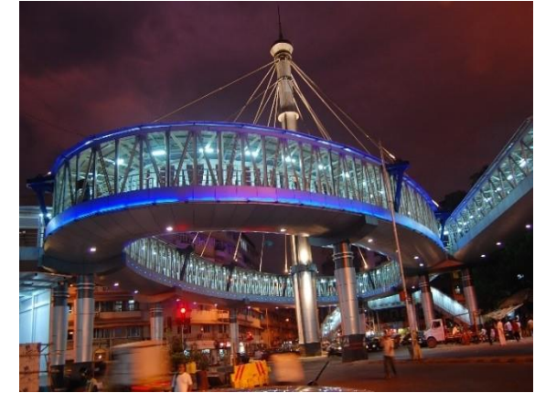
Grant road Skywalk
