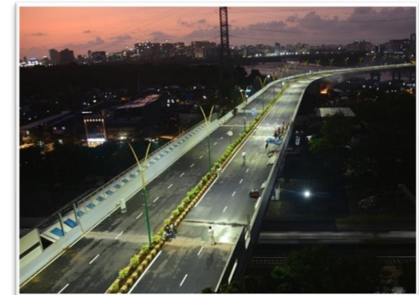
BKC- Chunabhatti Flyover
