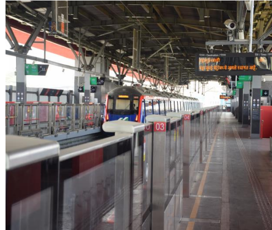
Mumbai Metro Line 7
