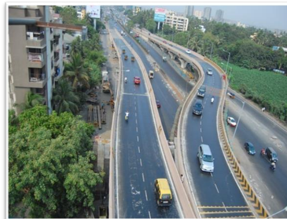
Amar Mahal Flyover
