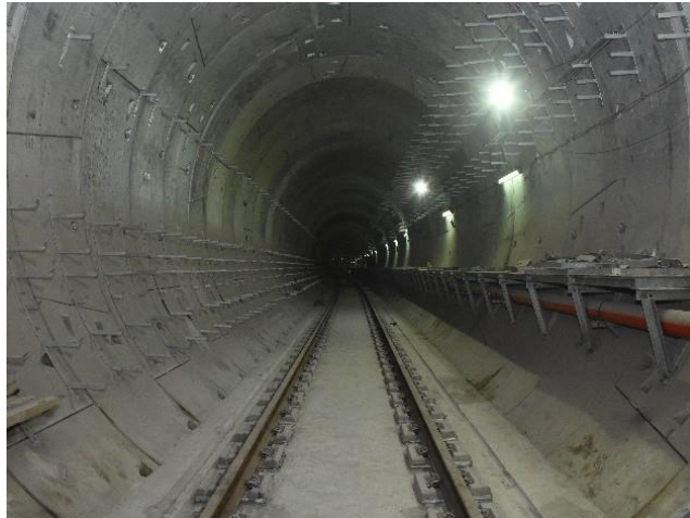
Mumbai Underground Metro Line 3
