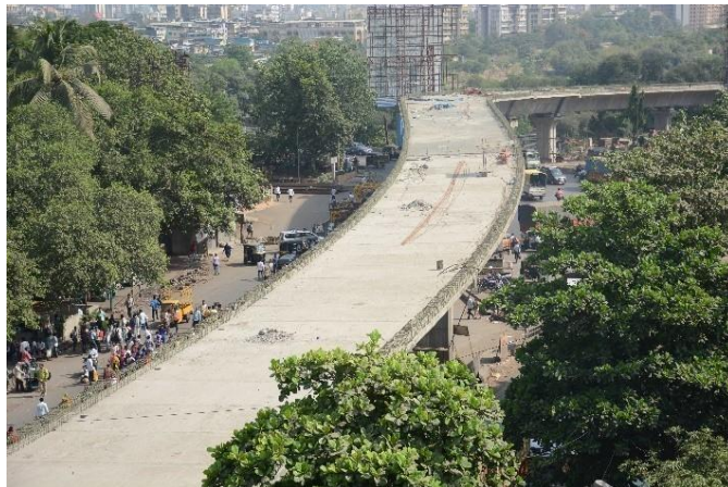
Kalwa Bridge Thane
