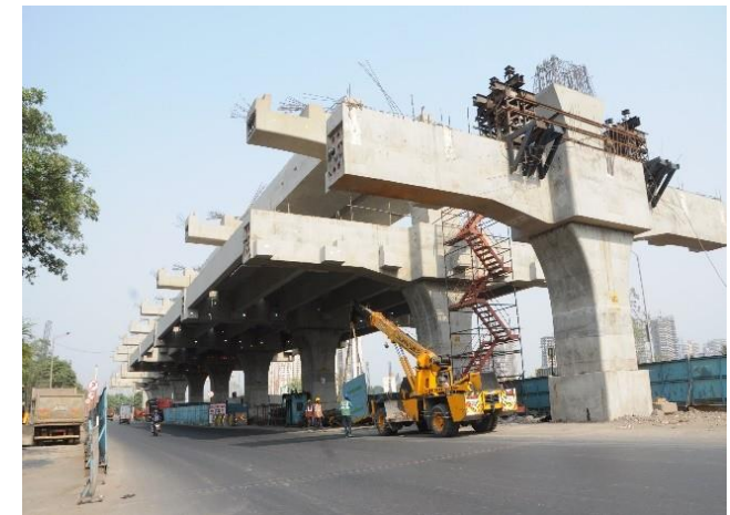
Mumbai Metro Line 6
