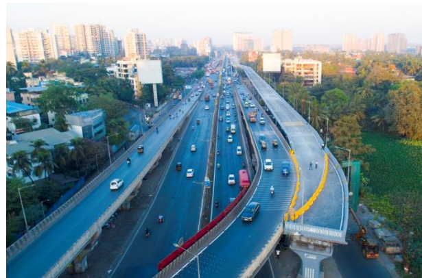
Chheda Nagar Flyover Part 1
