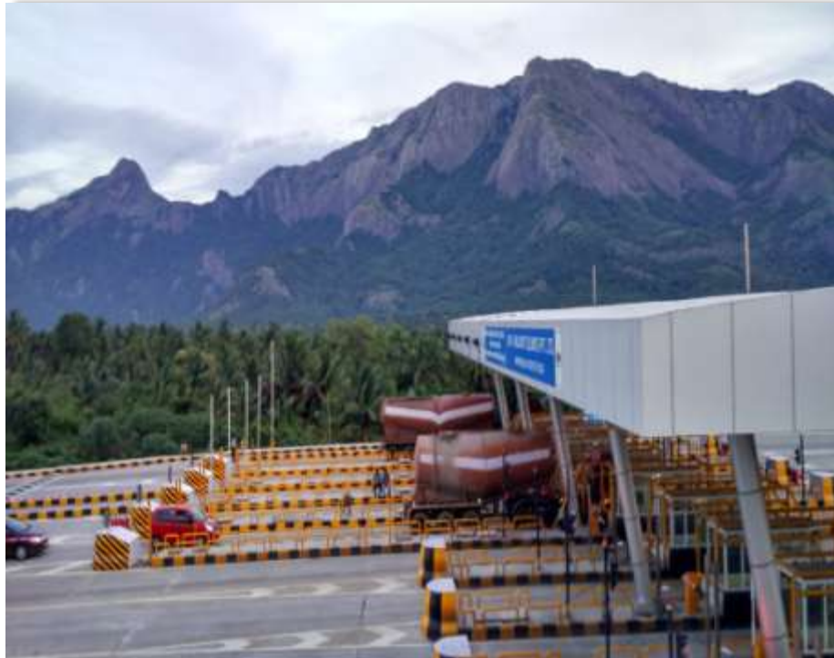
Walayar –Vadakkancherry BOT (Toll Road ) Project, Kerala
