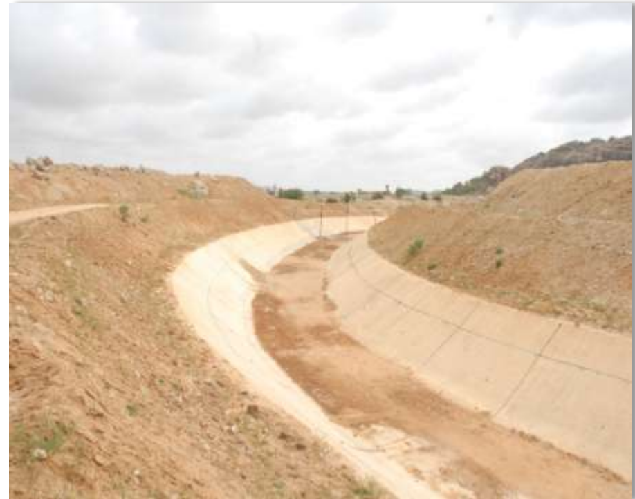
Irrigation Project in Telangana State
