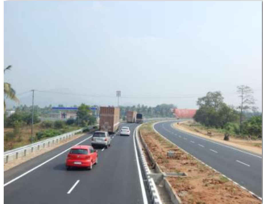
Walayar –Vadakkancherry BOT (Toll Road ) Project, Kerala
