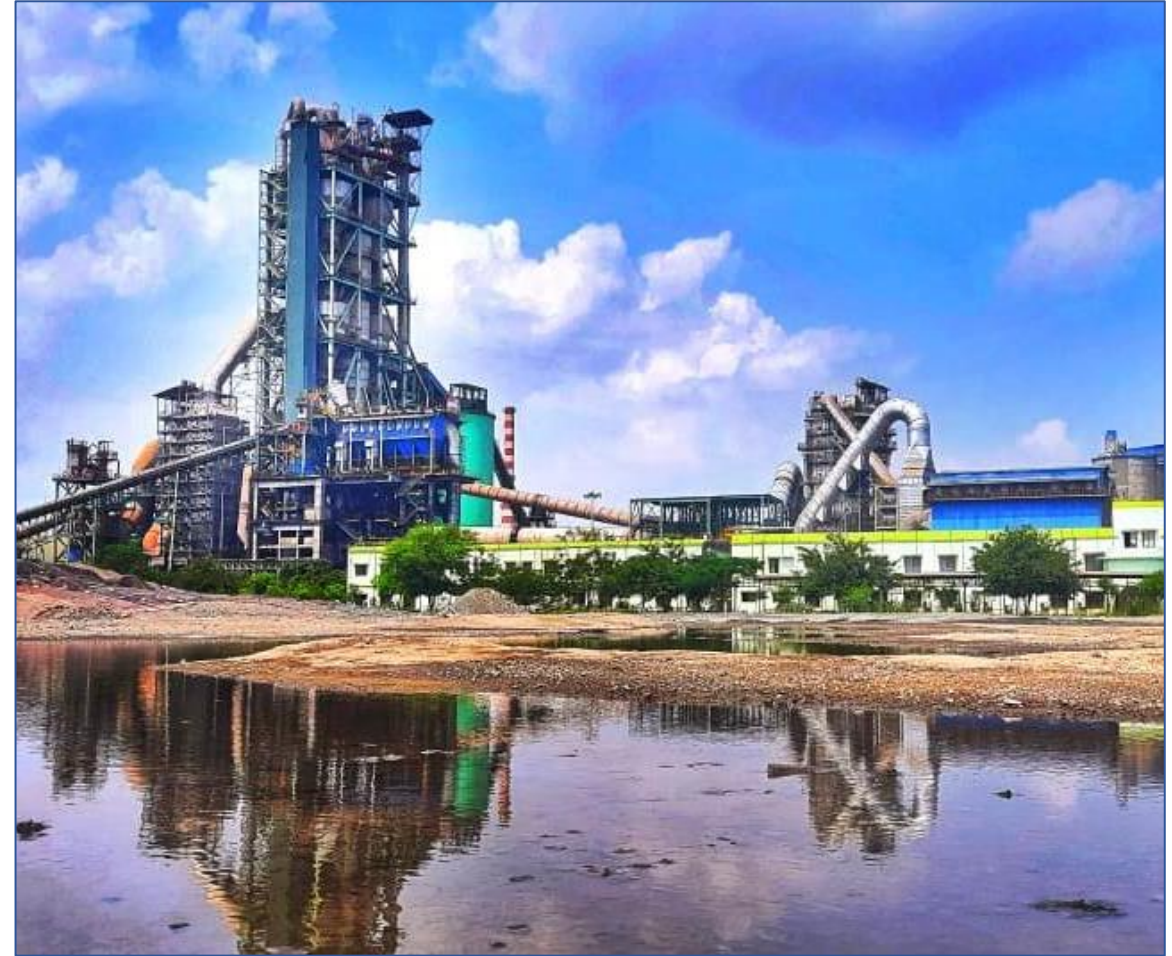
Chittor Cement Plant
