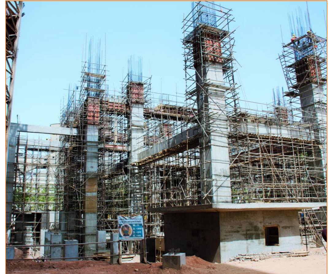
Roller Press building – Nimbol Debottlenecking project
