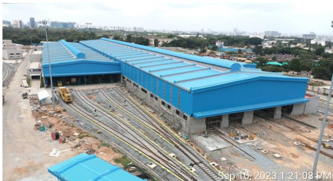
BMRCL (METRO SHED) - BANGALORE
