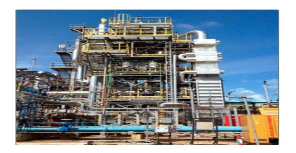
Power generated by using flu gases and capturing of heat through waste heat recovery boilers
