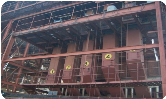
Bagasse Silos & Feeders of Boiler
