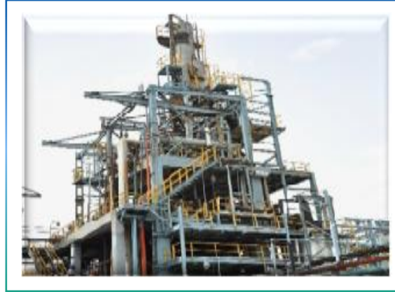
Chloromethanes plant, Mettur, Tamilnadu
