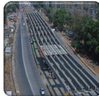
Mahape Flyover, Mumbai
