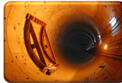
DMRC CC-24 Tunnel
