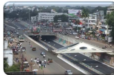
Grade Separator, Pune
