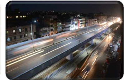
Flyover at Dhanakwadi
