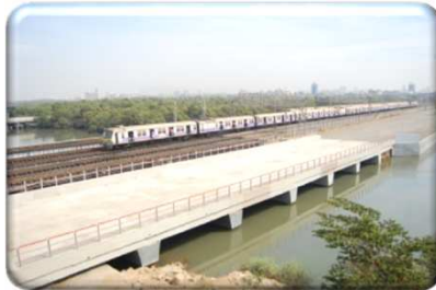
Bridge at Bandra -Mahim
