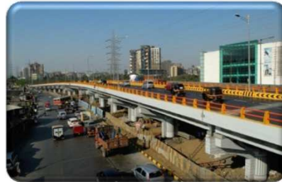
Flyover at Dindoshi, Mumbai
