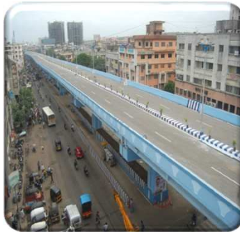
Dhankawadi Flyover, Pune
