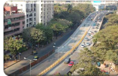
Flyover at Hindmata
