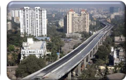
Flyover at Panjarapole, Mumbai
