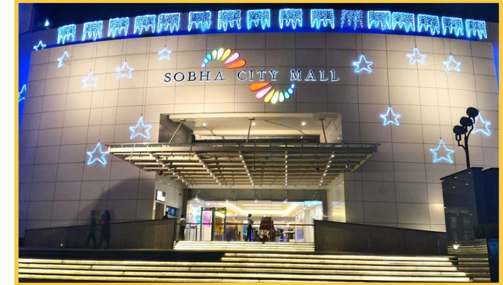
Sobha City Mall, Thrissur
