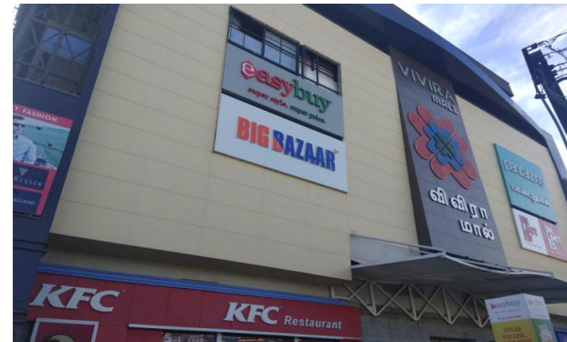
Board Façade Coverage mall Chennai HD
